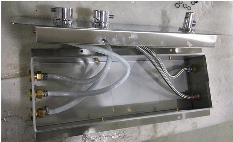
Inside of concealed box , it's so easy to repair , just take out the front of plate
